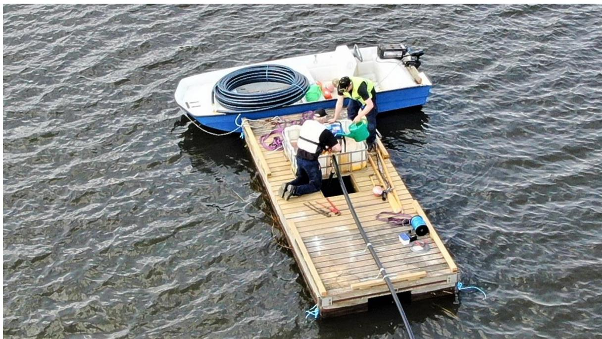
Figure 3. Installation of the irrigation pump at the raft.
